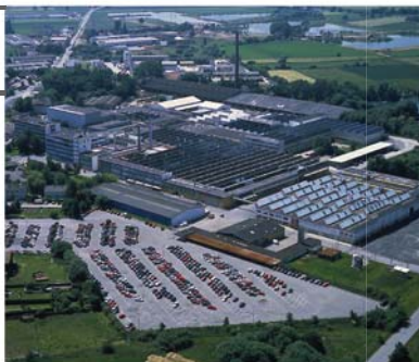
Stiebel Eltron's plant in Holzminden, Germany.
